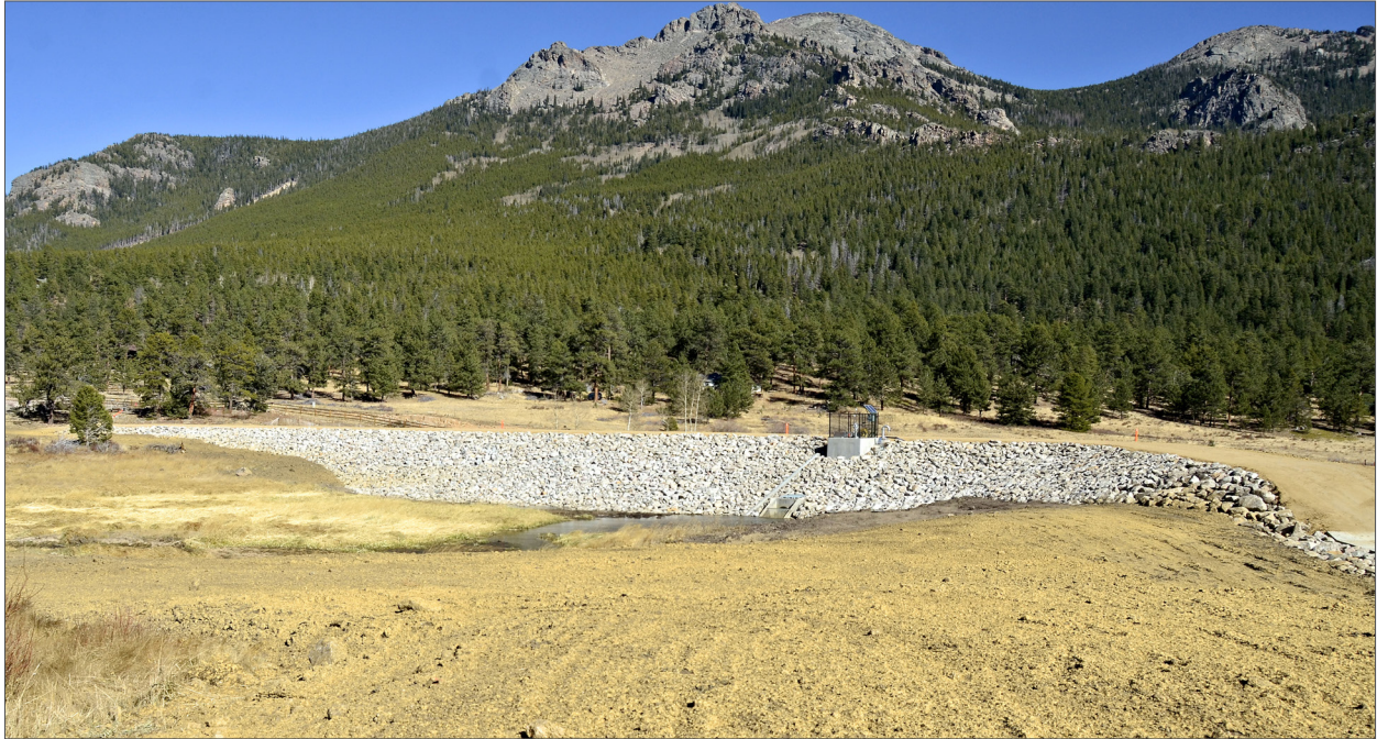
High Peak Camp Dam No. 4 (Continued) Estes Park, CO
